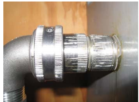
Figure 4: Assembly of Fittings onto Potted Nipple
